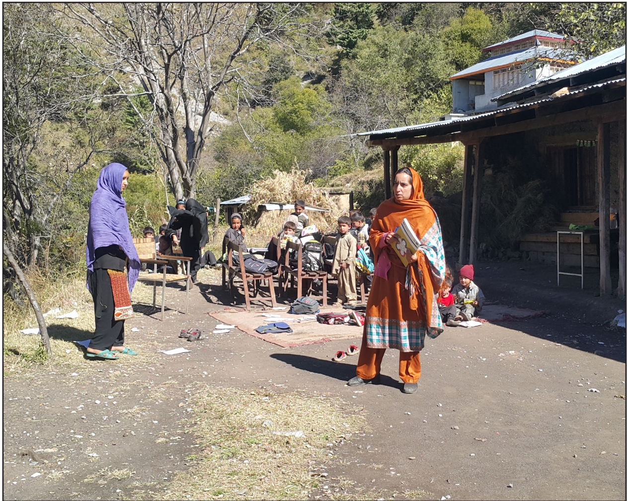
Thousands of schools in KP province like this one have been waiting for reconstruction since the 2005 earthquake, despite billions in international assistance.
